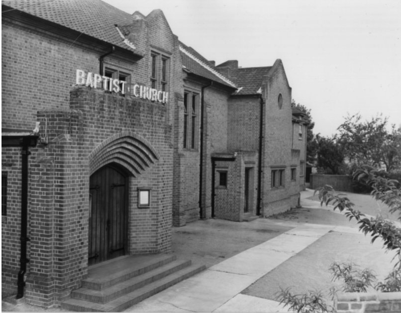
New Church building opened in 1940
